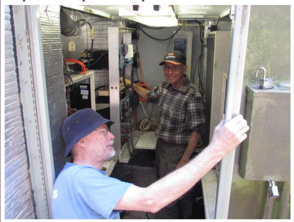
Picture shows Bernie N6FN (back) and Glen Al6RR (front) with initial installation of the rack components and DC power wiring. The 19" equipment rack on the left contains two 48 V to 13.8 VDC switching power supplies, SCOM controller and packet simplex repeater equipment.
